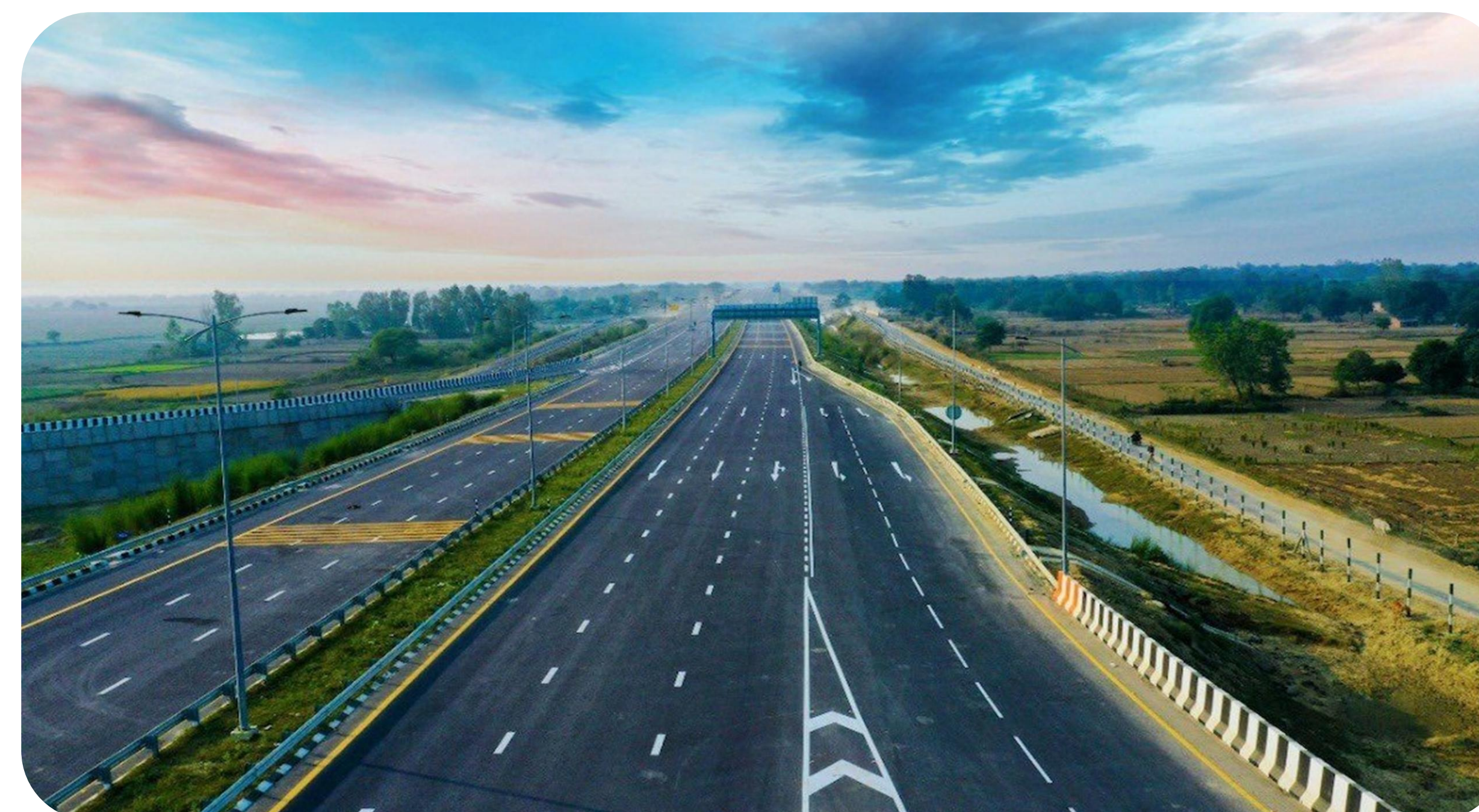
NEAR TO PURVANCHAL EXPRESSWAY
