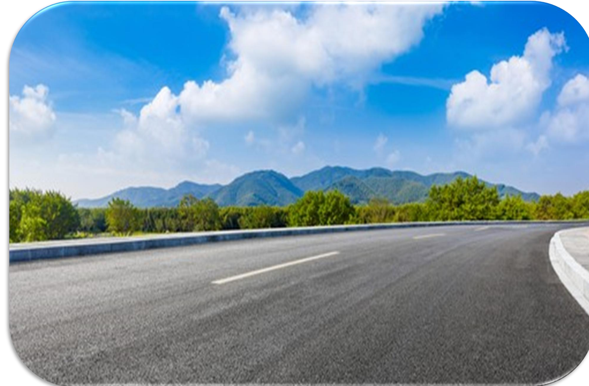
Wide Road with drainage system as Per LDA Norms
